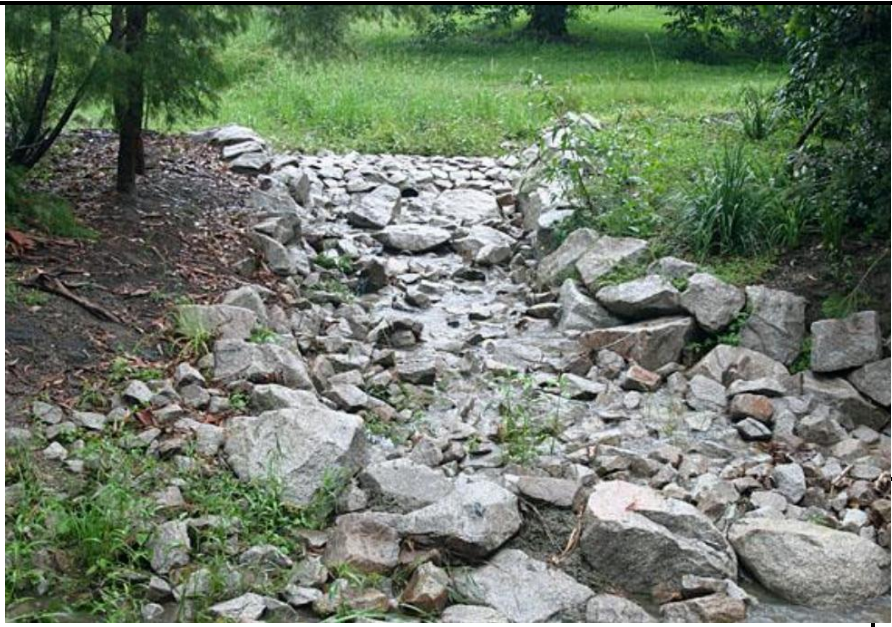
Example of buffered outfall with coarse aggregate (Catchments and Creeks Pty Ltd., 2020)
